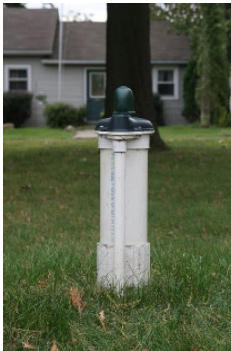
Private water supply well. Photo Credit: Iowa Department of Natural Resources (DNR)
